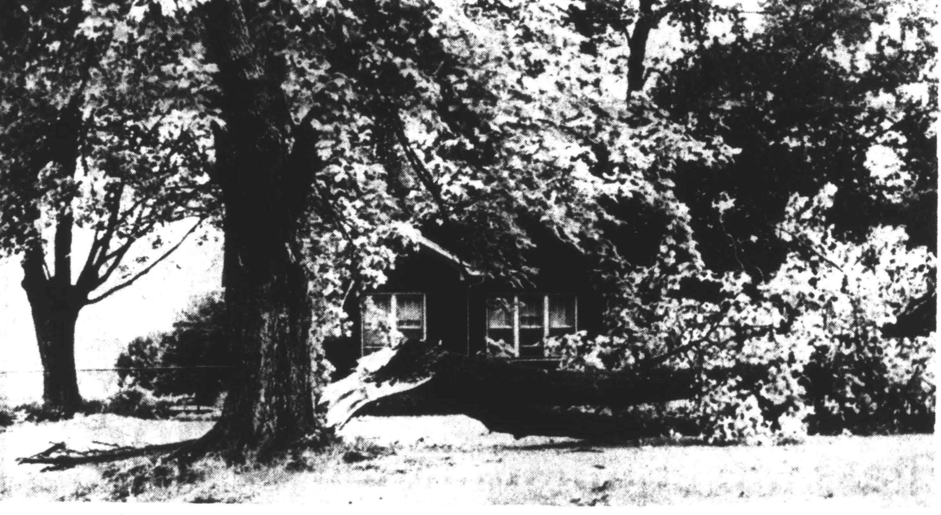
DAMAGE WAS CONFINED to trees and limbs late Monday afternoon as high winds struck Halls. Limbs from a tree on the First Christian Church lawn blocked South College Street, a black locust tree was uprooted in the backyard of Mr. and Mrs. Dave Strong and limbs blown from another tree, a tree was split on the lawn of Mr. and Mrs. David Nunn on West Main and limbs were strewn on almost every lawn in town. The roof of the E. G. Parker, Jr. building, next to the railroad in Gates, was badly damaged but property damage reported was minor.
